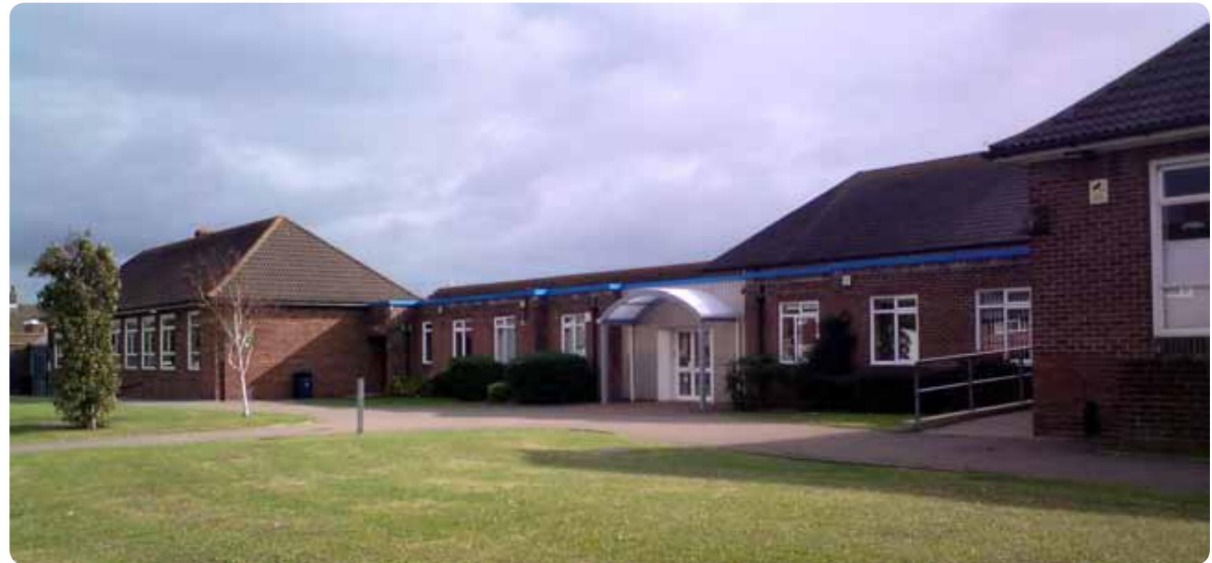
Existing Main Entrance
