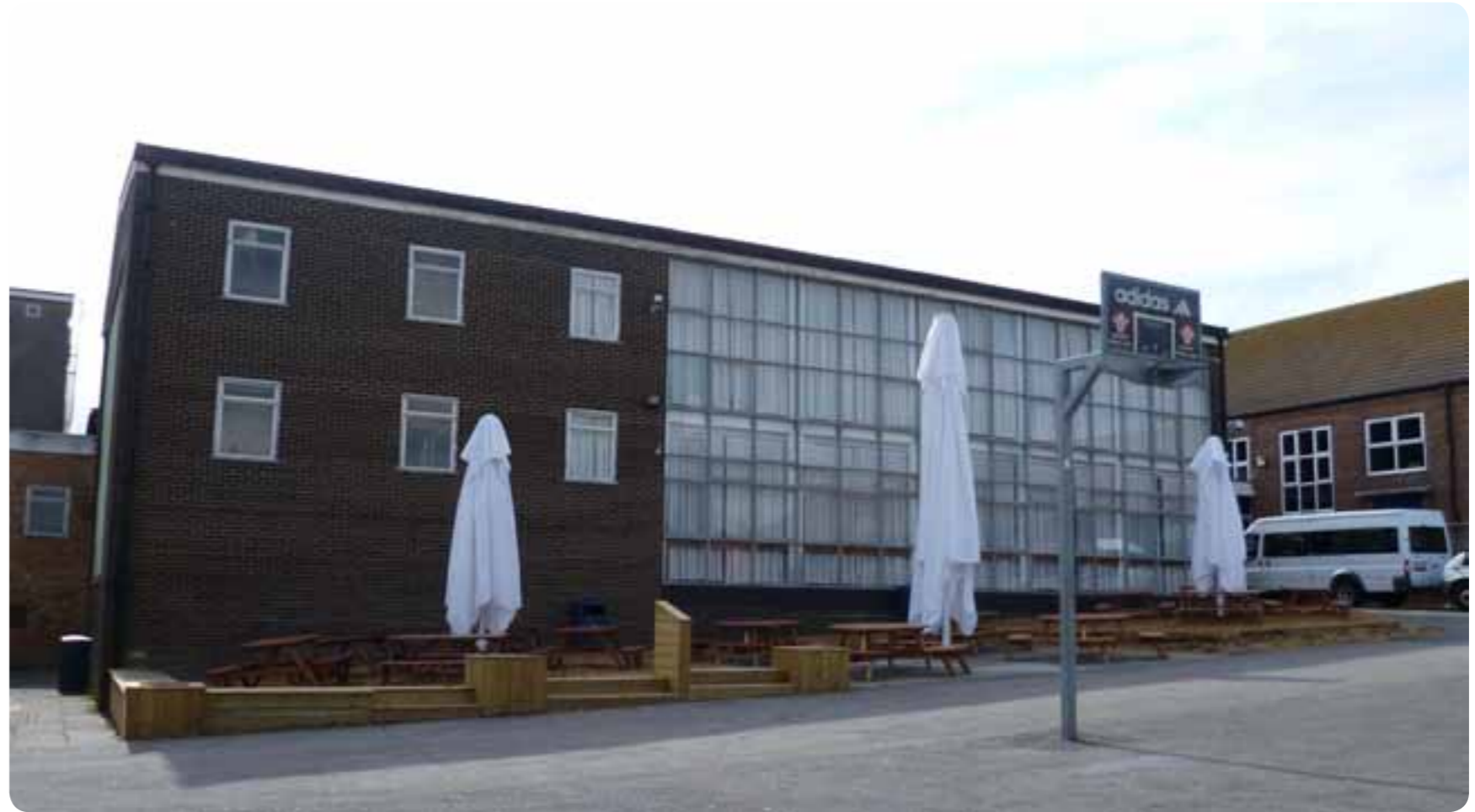
Existing hall, East elevation; with new decking and parasols
