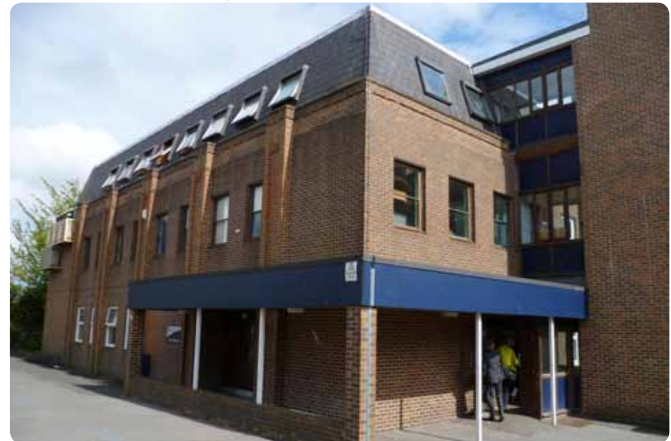
View of the Octogan building north elevation
