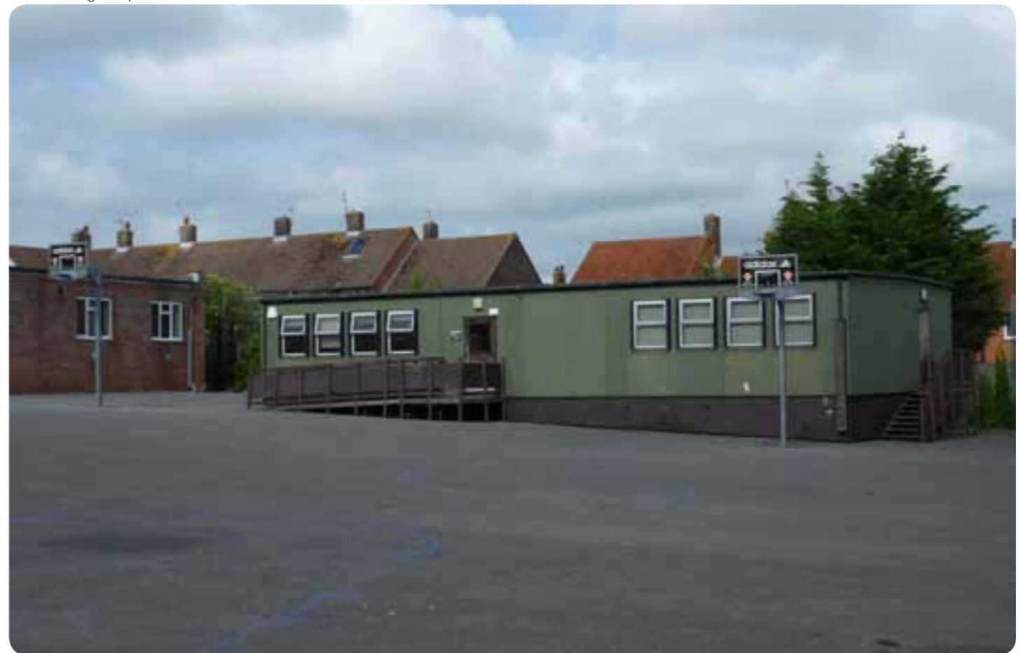
Existing mobile block on Eastern boundary; roofs of Henfield Road properties beyond
