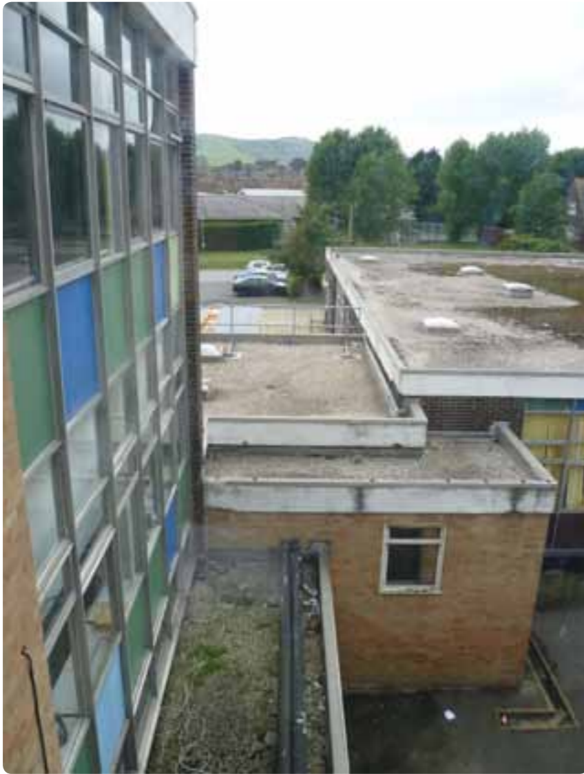
Poor quality existing fabric; hills beyond to the West
