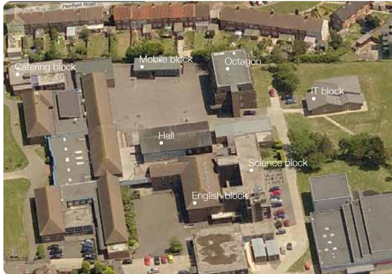
Existing site from the West
