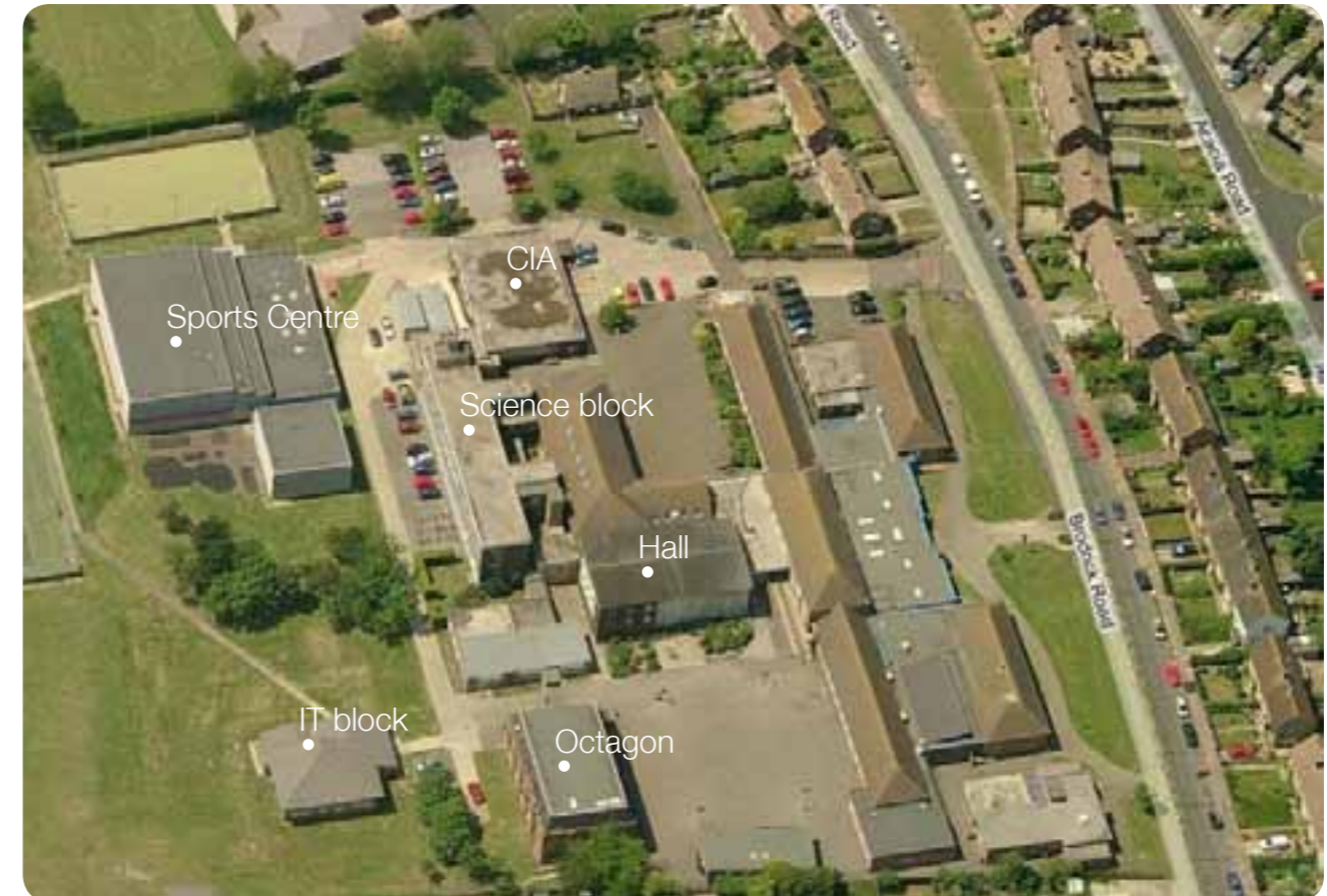
Site from the East
