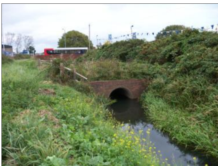
Plate 10: Bridge 5 of Phase 3 cycleway, looking northeast
