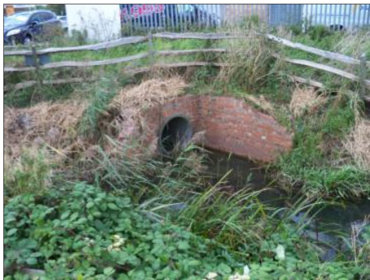
Plate 9: Culvert 2 of Phase 3 cycleway, looking north
