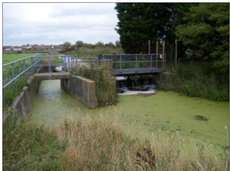
Plate 16: Weir-like structure beside Field 2 of Phase 3 cycleway, looking northeast
