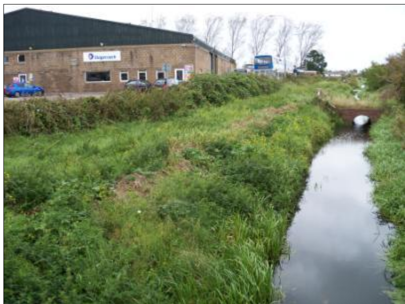
Plate 7: Phase 3 cycleway from Birch Road, looking northeast
