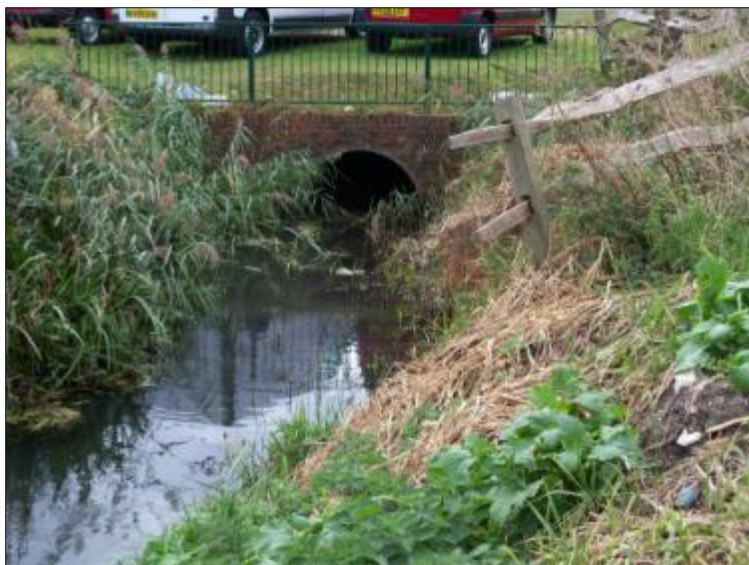
Plate 8: Culvert 1 of Phase 3 cycleway, looking southwest
