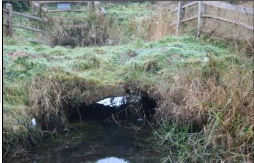
Plate 5: Bridge 4 of Phase 2A cycleway
