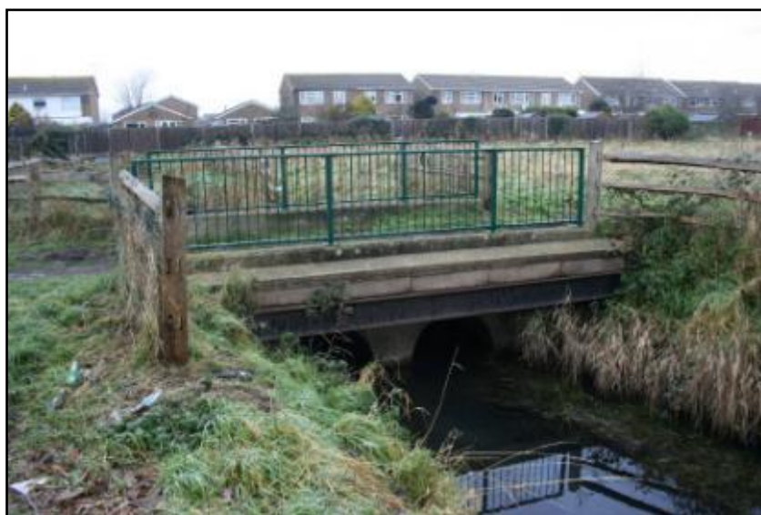
Plate 3: Bridges of Phase 2A cycleway (Top: Bridge 1; Middle: Bridge 2; Bottom: Bridge 3)
