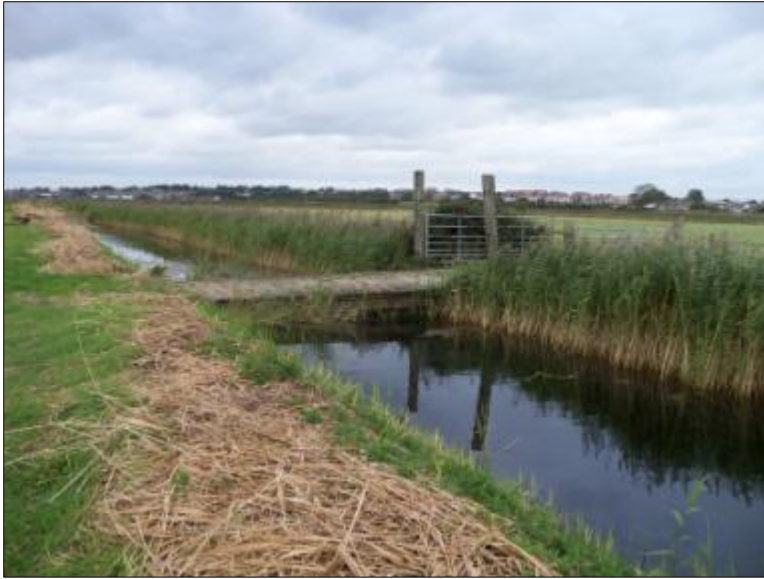
Plate 17: Bridge 8 of Phase 3 cycleway, looking north
