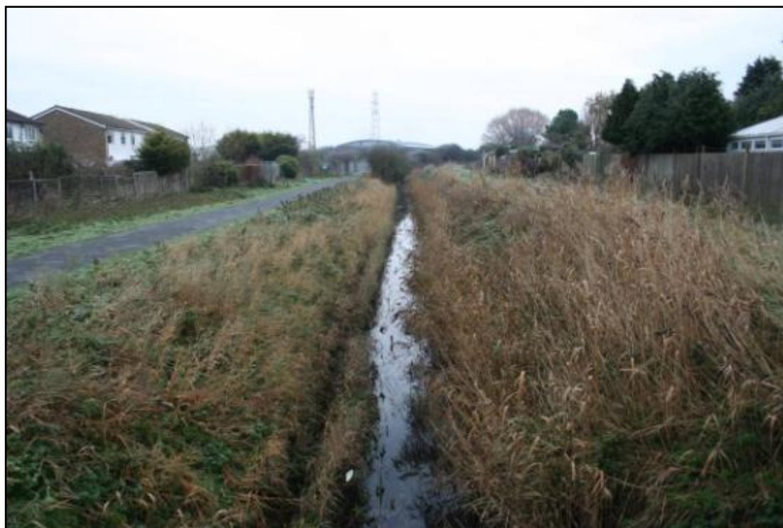
Plate 2: Horsey Sewer along Phase 2B cycleway, looking northeast from Churchdale Road
