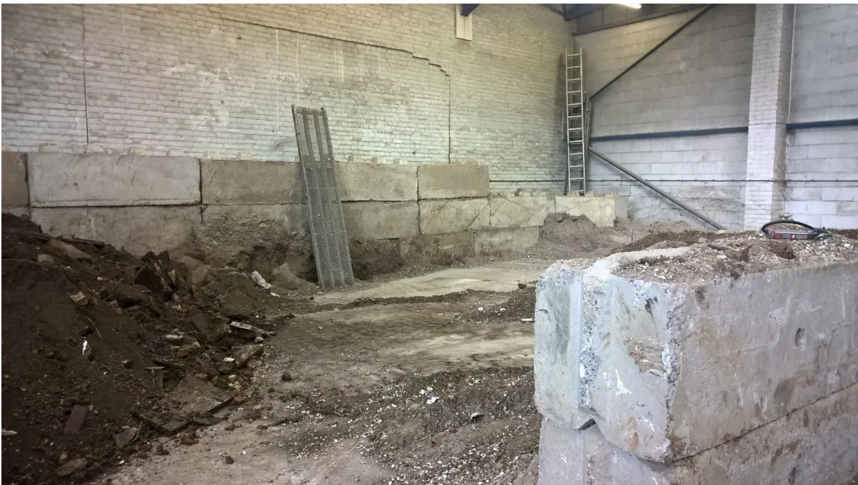
Figure C6– Photograph illustrating the concrete bunding blocks currently in use at the existing site which are to be utilised at the proposed site's northern boundary.
