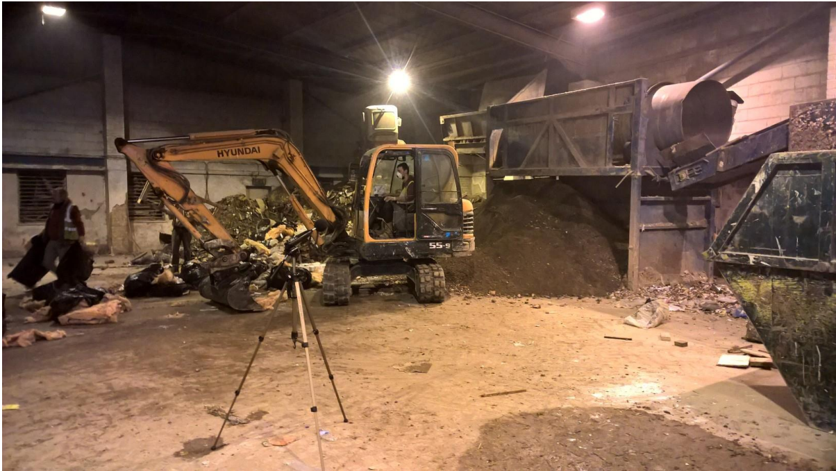
Figure C5 – Photograph illustrating a measurement position at the existing Greenacre site. The trommel, 2 tonne excavator, 5 tonne excavator are in simultaneous operation.
