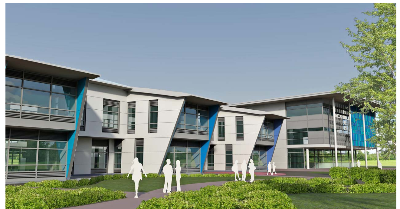
View of Eastern elevation
