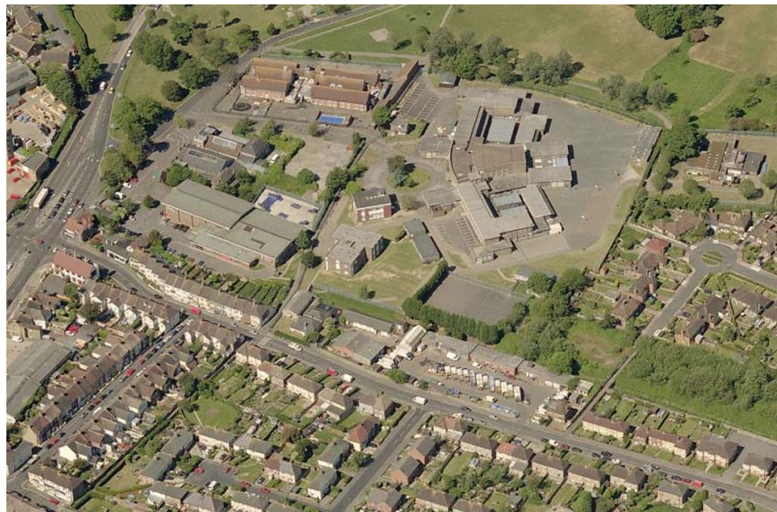
Existing School at the Down Road site
