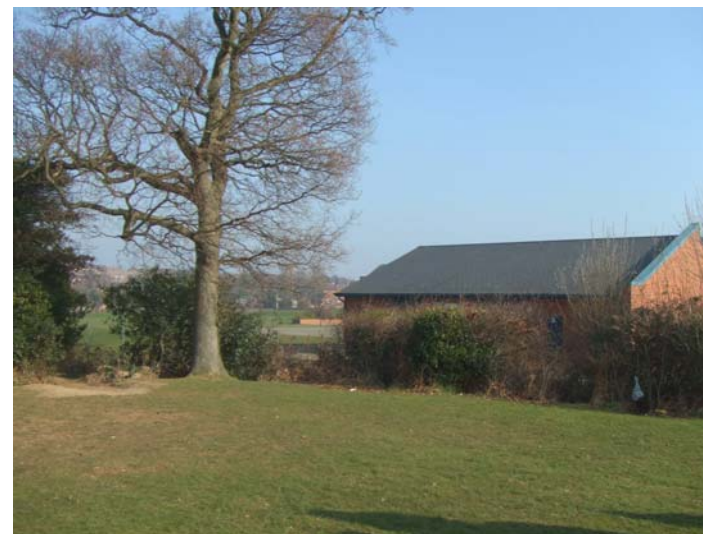
View of existing building from site
