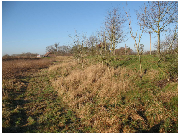
Photograph 6 : Bund looking south
