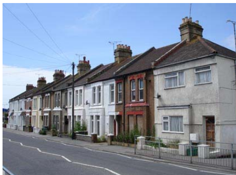
Photograph 17 East Elevation of London Road Buildings
