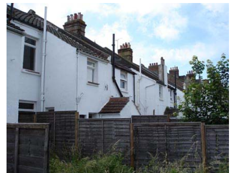
Photograph 18 West Elevation of London Road Buildings
