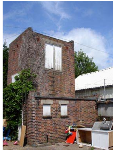
Photograph 20 Brick Tower to North of Nursery School
